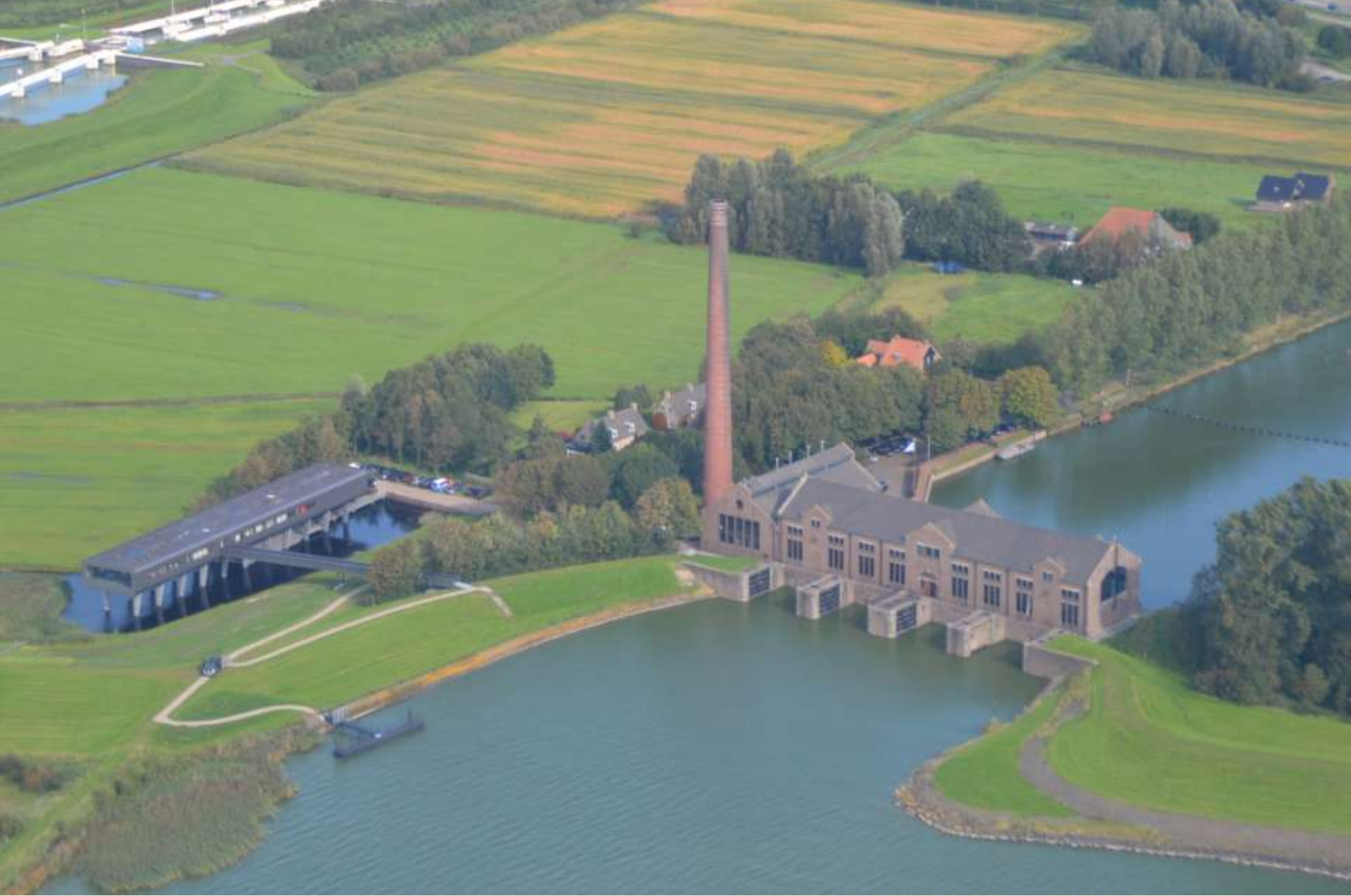
Ir. D.F. Woudagemaal / D.F. Wouda Steam Pumping Station (1998)
